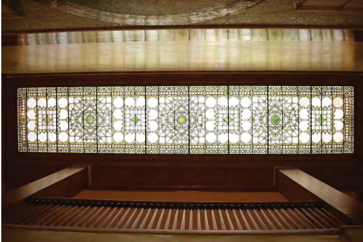
Photo 34. Main Stairs stained-glass laylight, view up.
