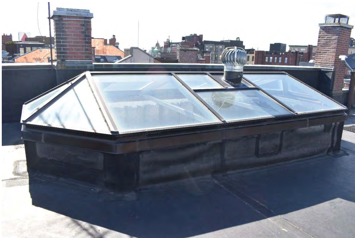
Photo 44. Elliptical Stair, rooftop structure, view southeast.
