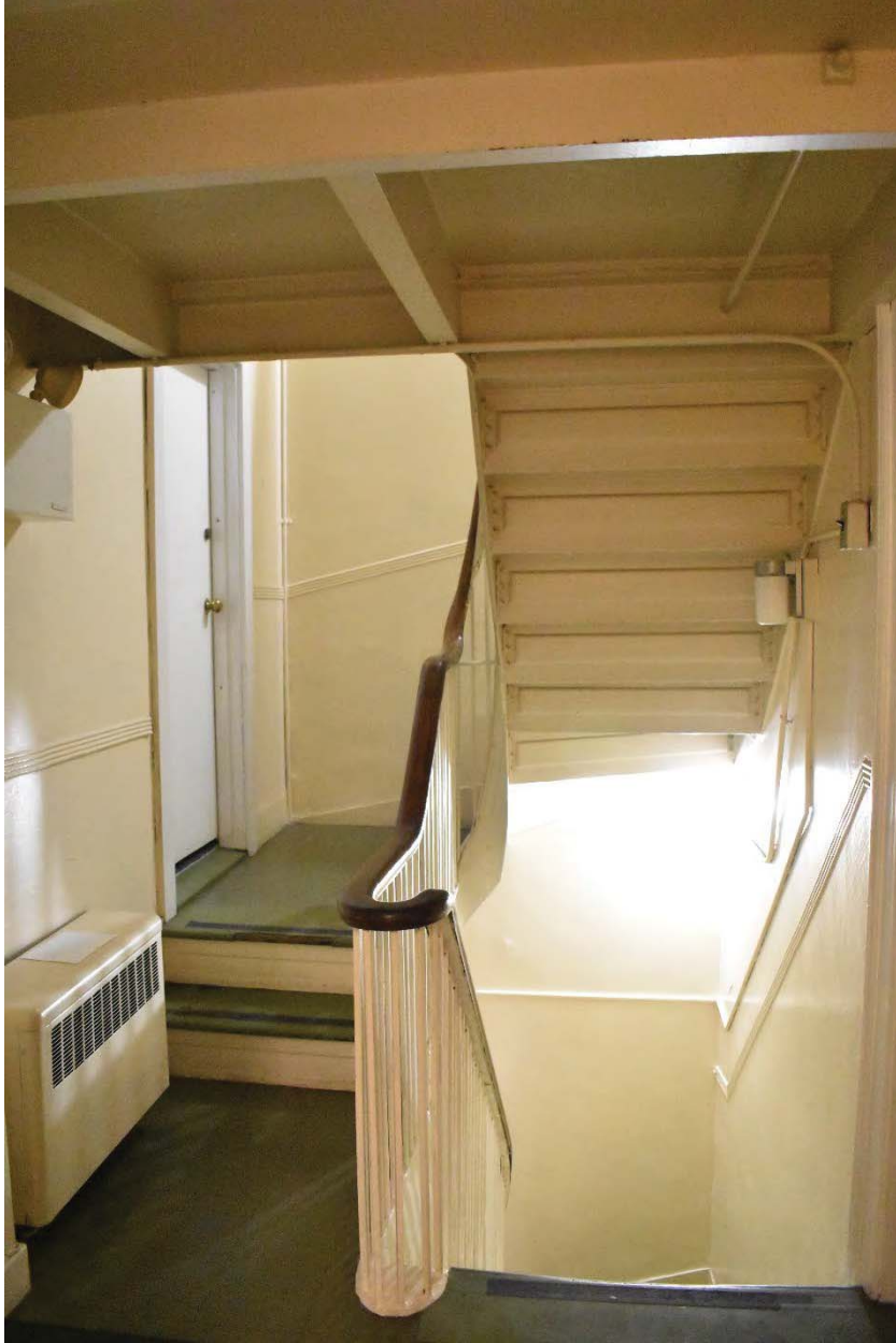
Photo 25. Service stair, view east.
