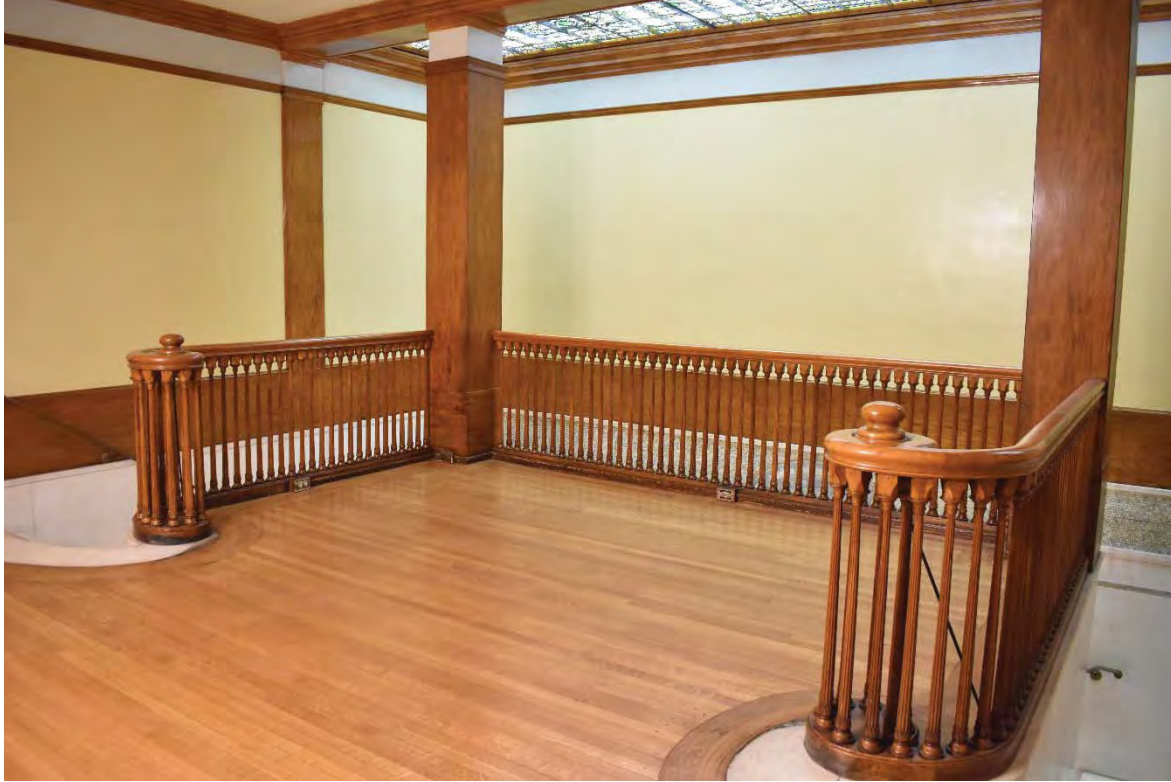
Photo 36. Stair Hall, view northeast.
