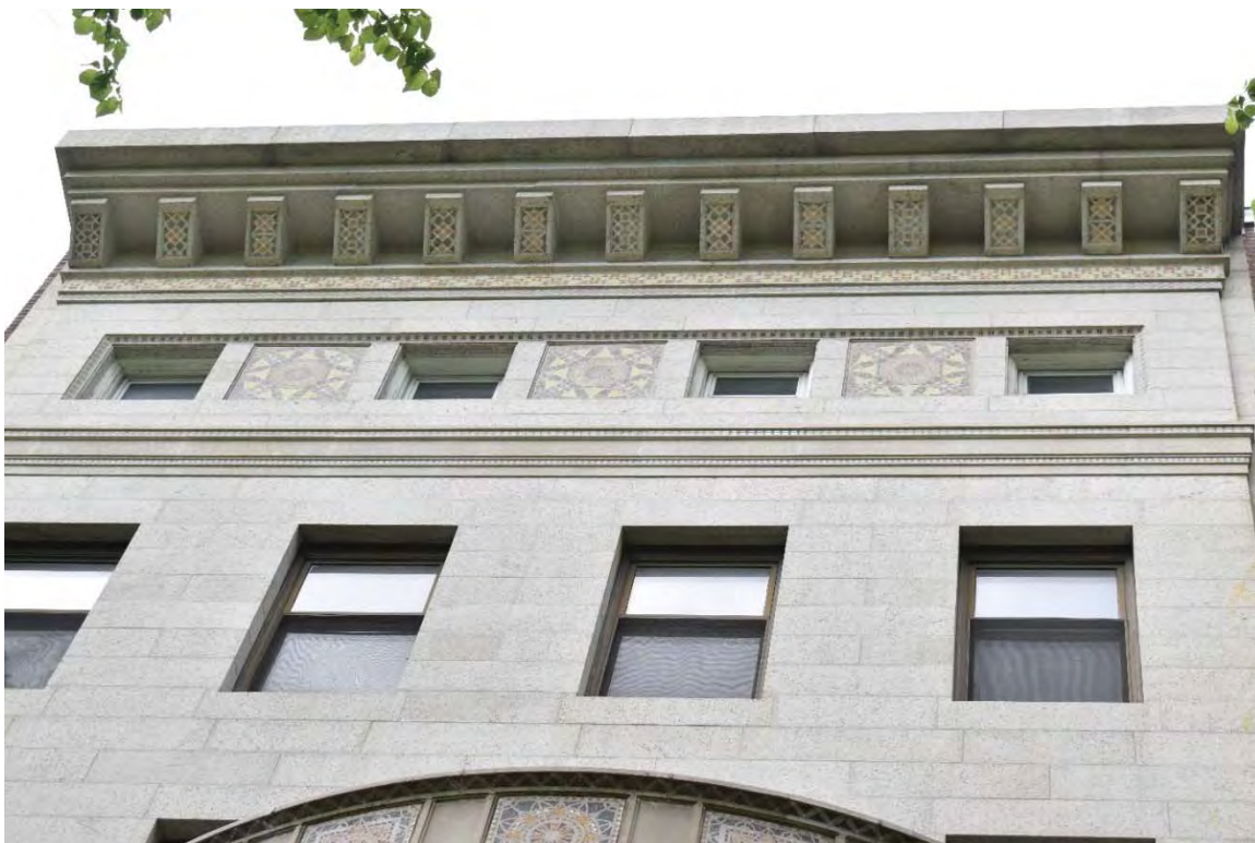
Photo 6. Facade, upper floors and cornice, view north.
