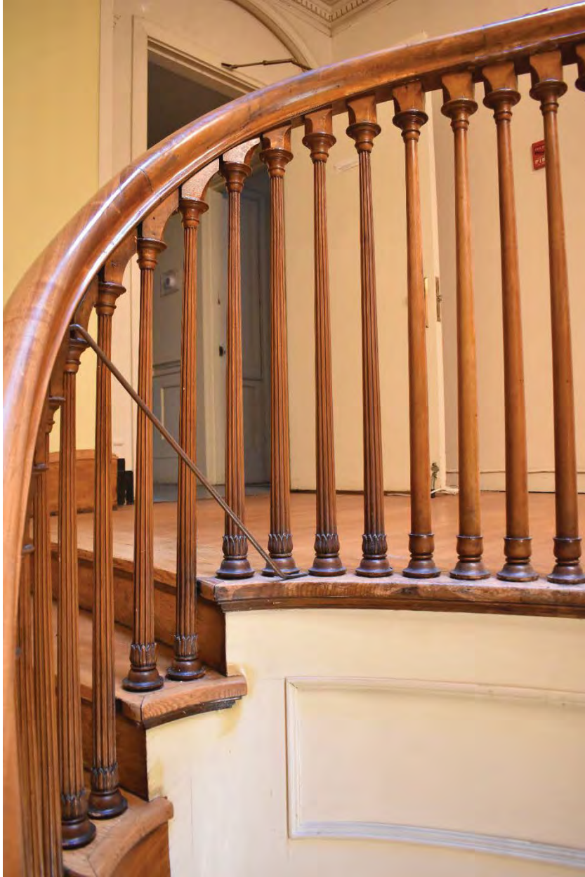
Photo 41. Elliptical Stair, view down.
