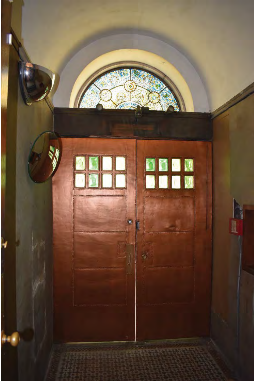
Photo 7. Outer Vestibule, main entrance doors, view south.
