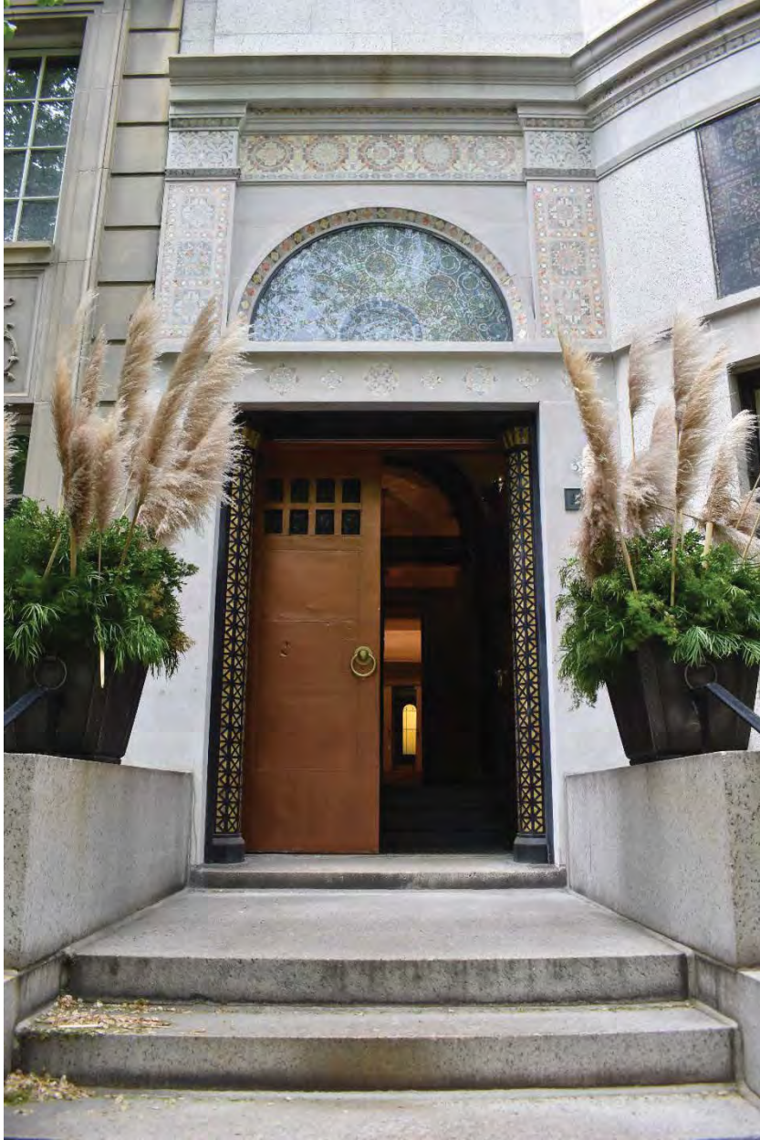
Photo 4. Facade, main entrance, view north.
