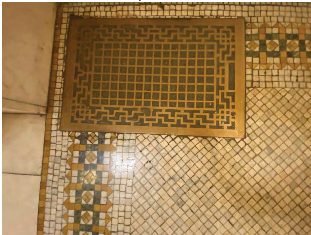
Photo 16. Marble Hall, floor detail, view down.
