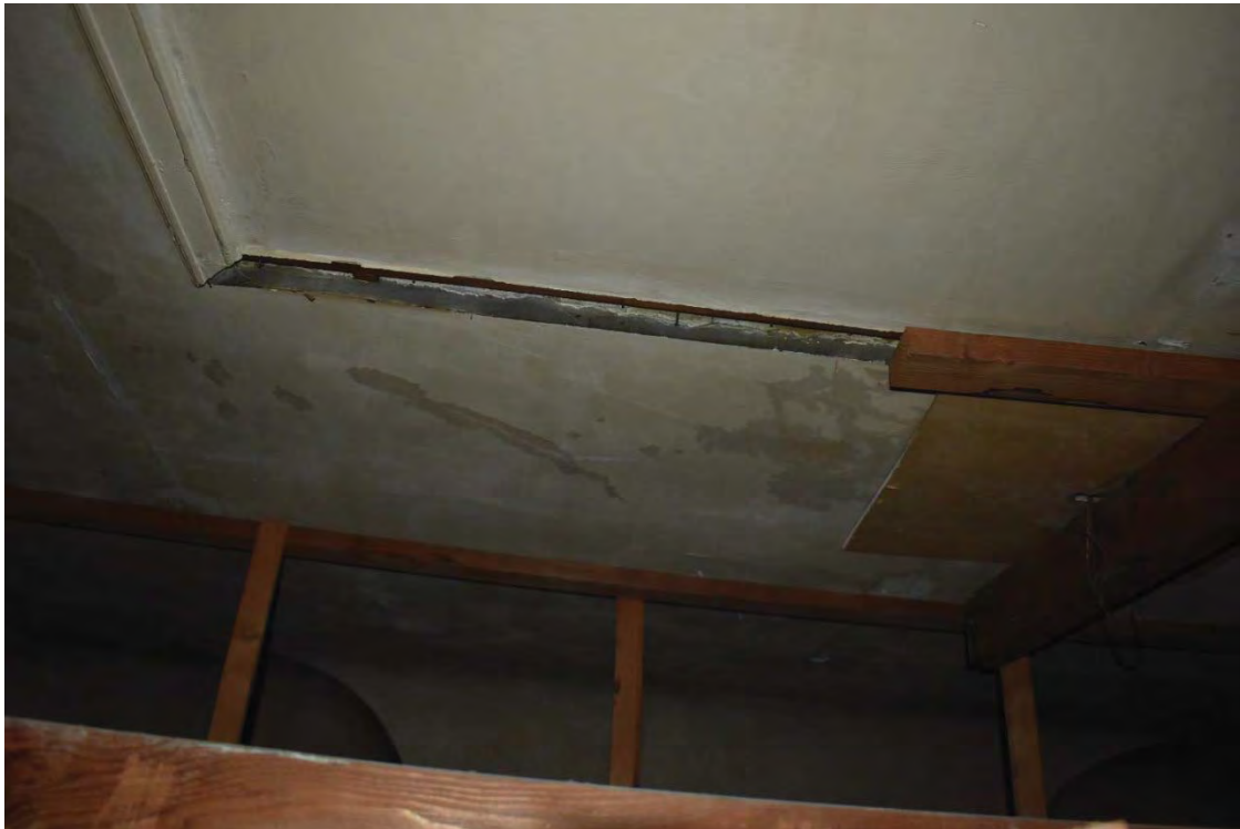
Photo 56. Sky Parlor, covered skylight, view up.
