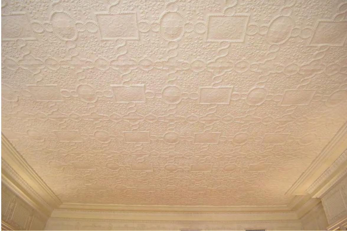
Photo 30. Drawing Room, ceiling detail, view south.
