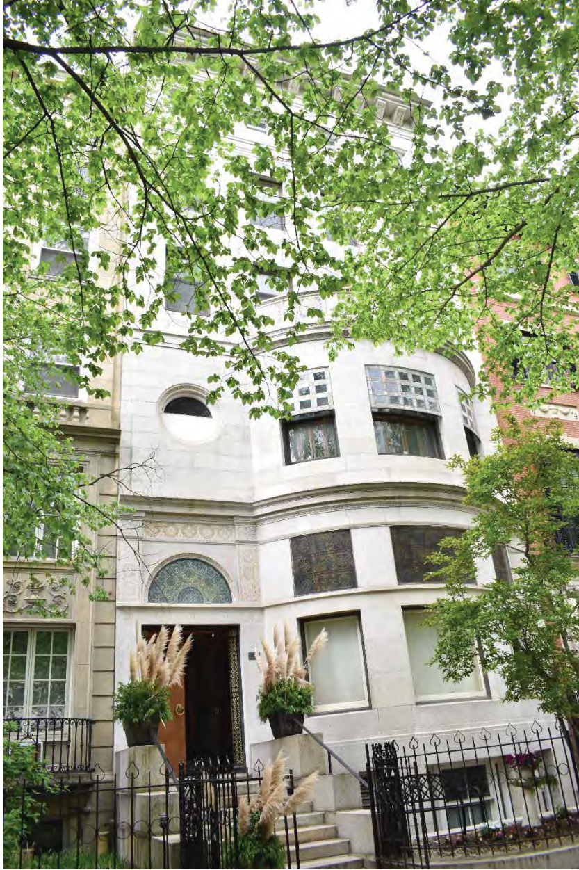
Photo 1. Front facade, view northeast.
