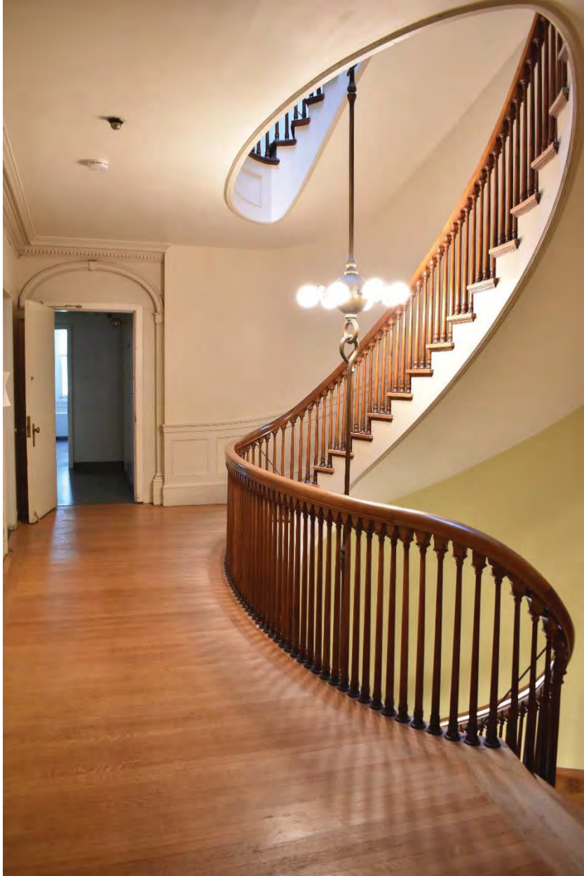
Photo 38. Elliptical Stair, third floor, view south.
