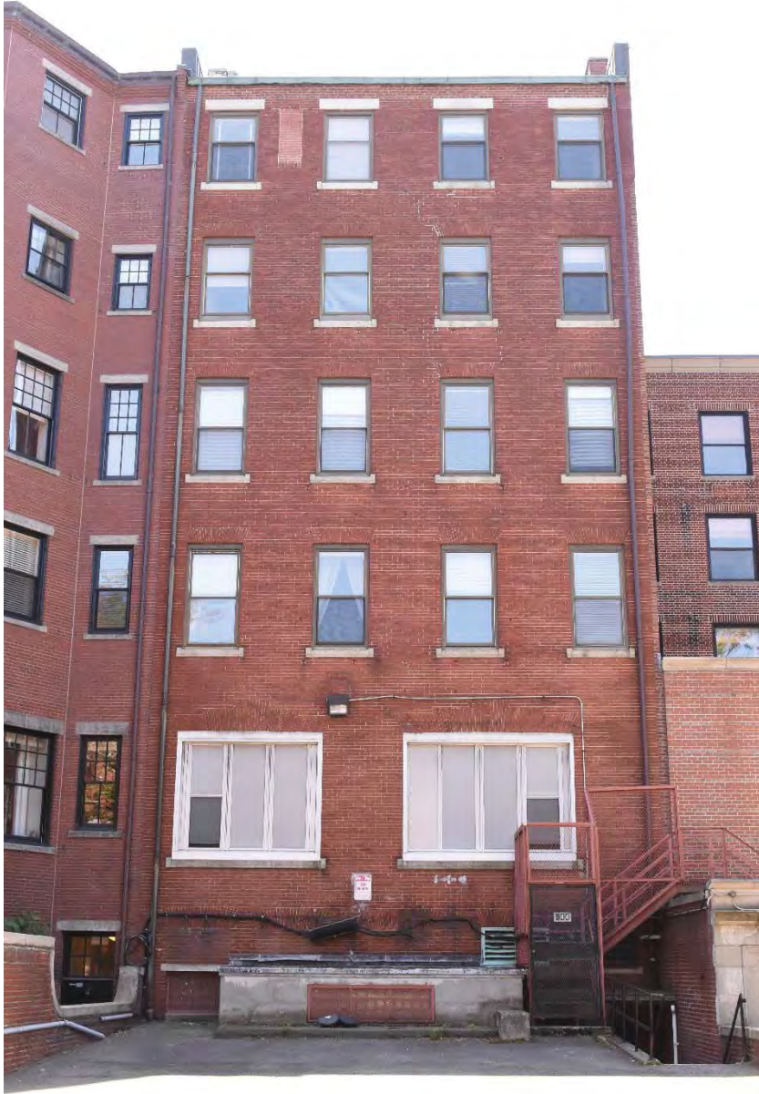
Photo 3. Rear elevation, view south.
