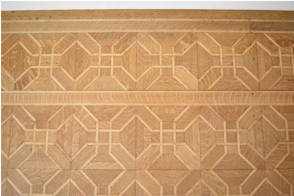
Photo 31. Drawing Room, floor detail, view down.
