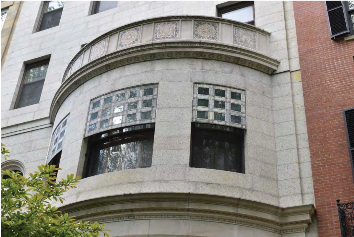
Photo 5. Facade, bow, view north.
