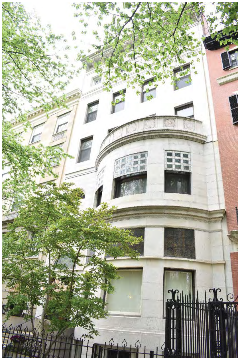
Photo 2. Front facade, view northwest.
